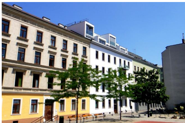
The house Odeongasse 11 located in a pedestrian zone
